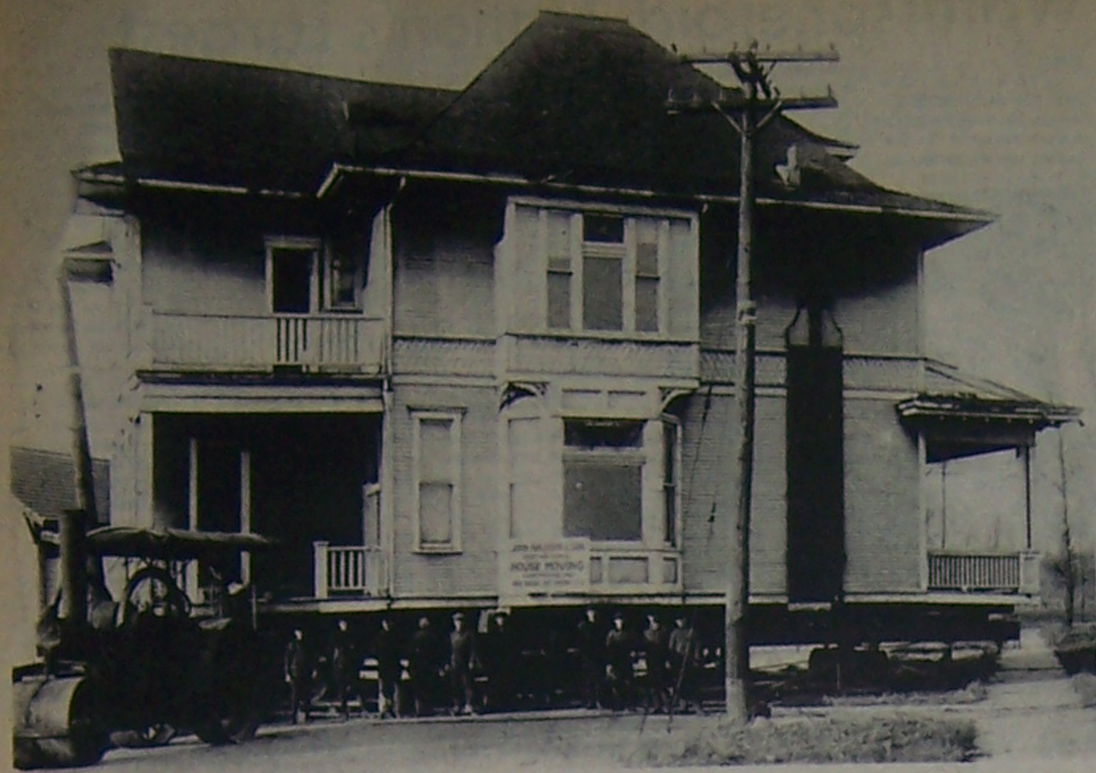
House movers brought many large homes across the State Line from Hammond in the early 1920s. One of the movers was the father of local contractor Zygmunt Jocha. 701 Memorial Dr., Calumet City. Jocha's father left the moving business in 1925 to establish his own construction firm.
